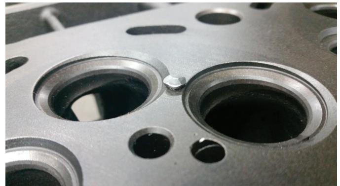
Lock-N-Stitch Repair Pin After Installation and Peening
